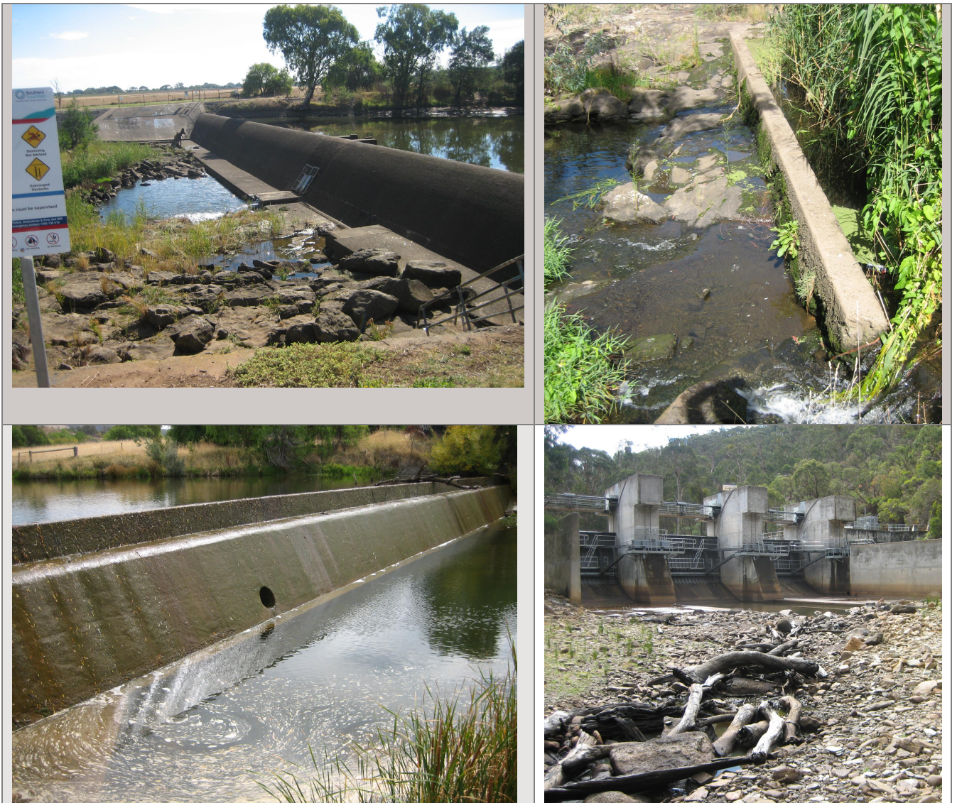
Figure 9-1: Examples of fish barriers in the Werribee River catchment. Top left – Lower Diversion Weir (Werribee); Top right – small concrete barrier downstream of Bungeys Hole; Bottom left – Upper Diversion Weir (Bacchus Marsh); Bottom right – Lerderderg Weir (this structure has a vertical slot fishway to assist fish passage).
