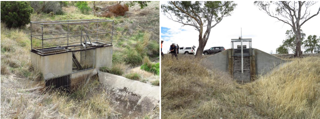
Figure 1-2 Left: Regulator structure at the inflow pipe from Green Lake to Dock Lake. Right: Regulator on the outfall channel from Dock Lake to Burnt Creek.
