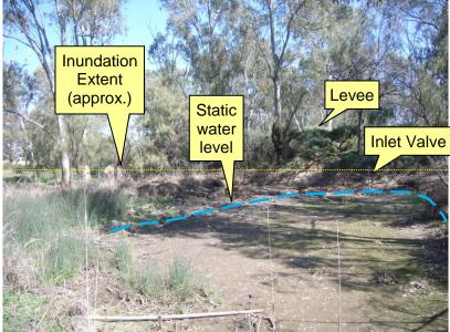
**Figure 22 The downstream end of Sandilong Creek, during drawn down** Key: Blue dashed line: Approximate static water level; Yellow dotted line: Approximate inundation extent. The Murray River is situated a short distance behind the levee bank. *Image: Sunraysia Environmental Pty Ltd.*
